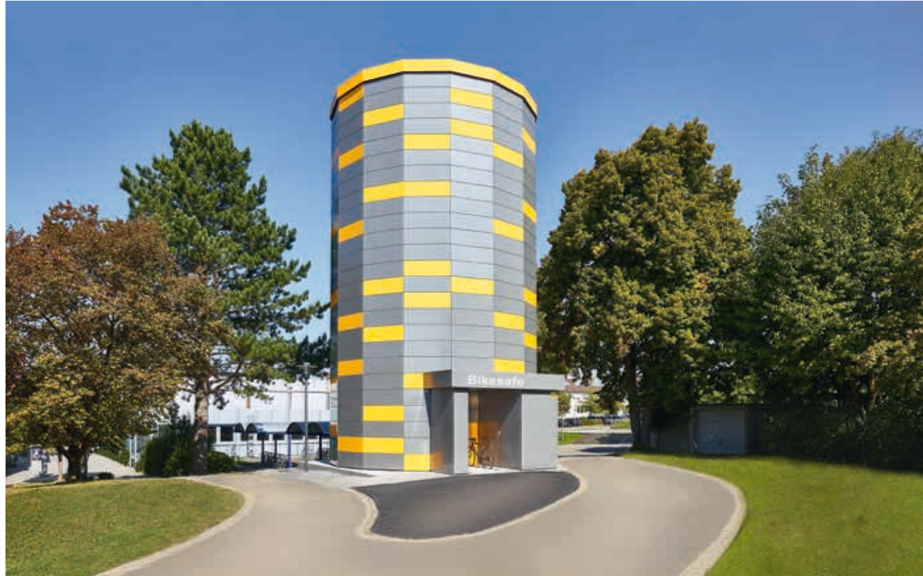
The tower version of the Wöhr Bikesafe accommodates 122 bicycles in the smallest of spaces.
