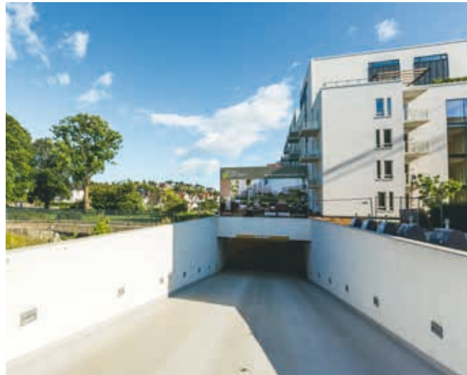
An approx. 8,000 m 2 underground car park with 250 parking spaces is located beneath the courtyard.
