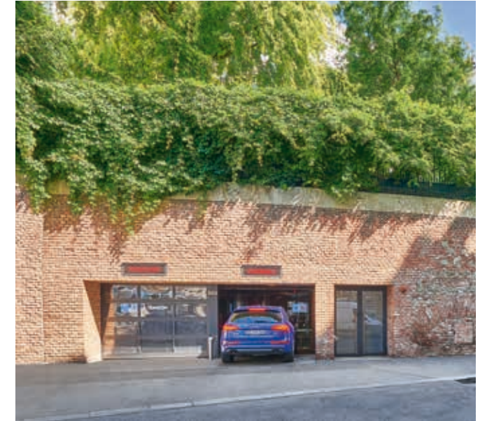
The entrance to the Wöhr Parksafes was integrated into the former garden wall.
