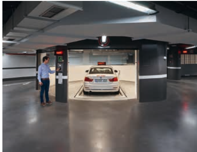
The system is adaptive: those who use their car frequently are allocated a space close to the drop-off and retrieval point.
